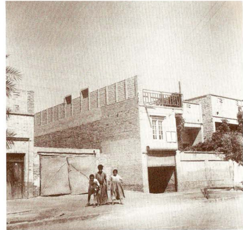
Fig. 54. Residence in Baghdad, Iraq, with two small malqaf openings high on the side of the buildings, as typical in regions with very hot seasons. (See p. 59.)
