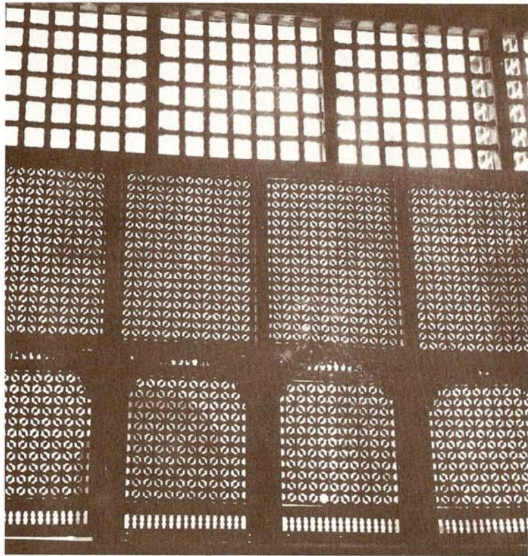
Fig. 23. Mashrabiya of the Jamāl Ad-Dīn Adh-Dhahabī house, Cairo, showing increased interstitial spacing at high levels. (See p. 48.)
